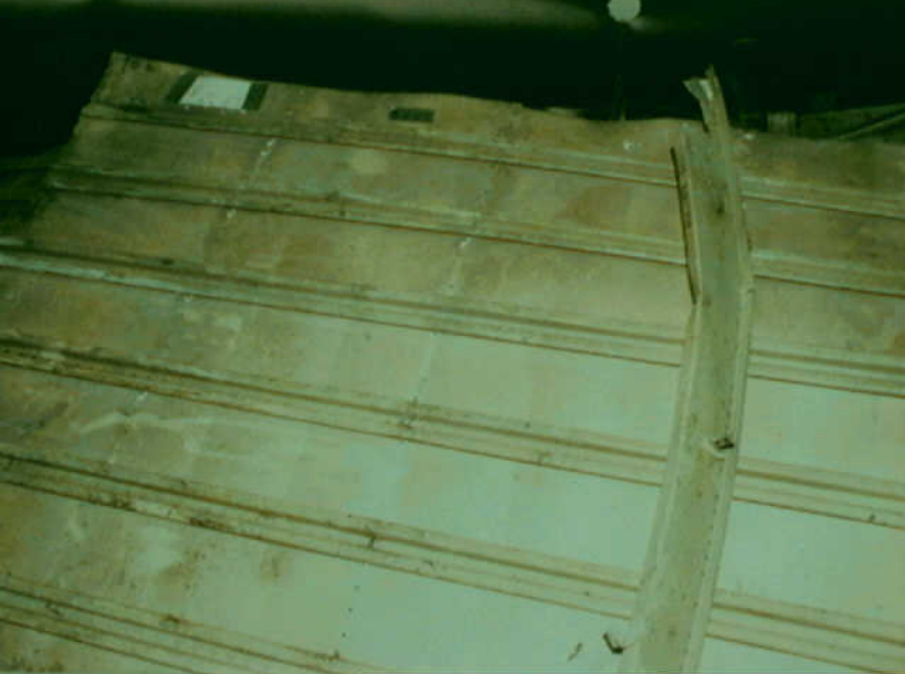
Structures 7 - LF39 - Photo 3
