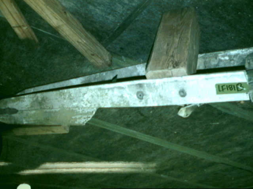
Structures 7 - LF181 - Photo 4
