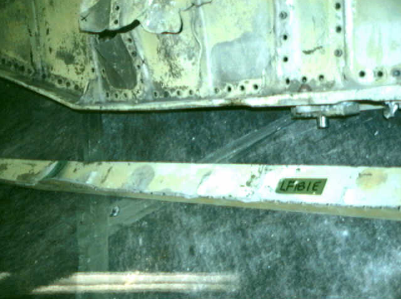
Structures 7 - LF181 - Photo 1
