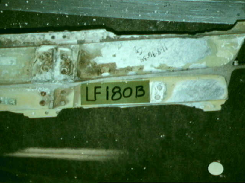
Structures 7 - LF180B - Photo 1
