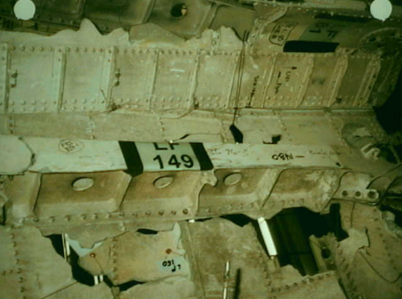
Structures 7 - LF149 - Photo 1
