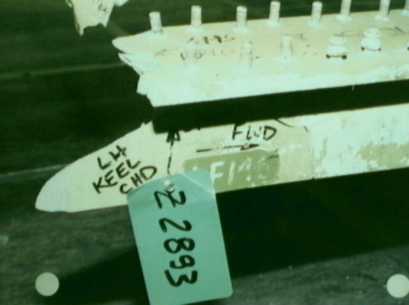
Structures 7 - LF14 - REV/ADD Photo 5
