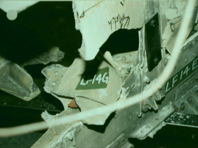
Structures 7 - LF14 - REV/ADD Photo 3
