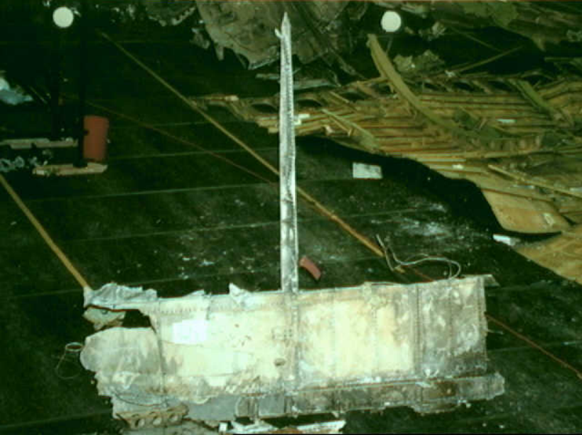
Structures 7 - LF14 - Photo 8
