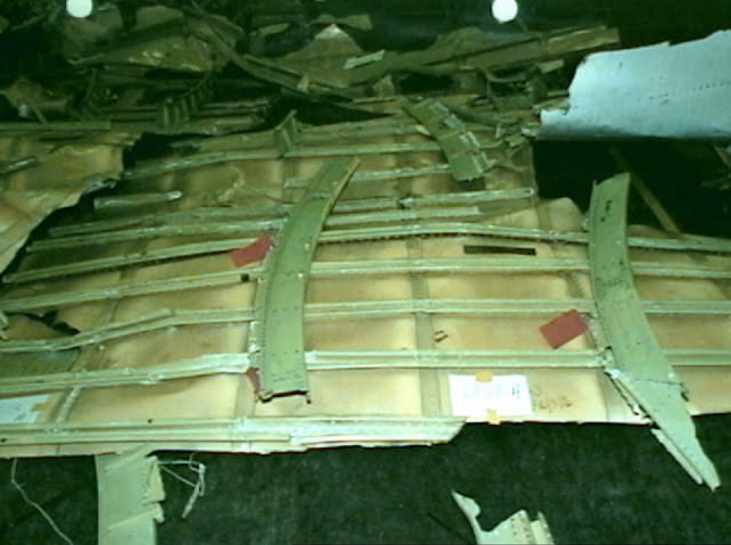
Structures 7 - LF13 - Photo 2
