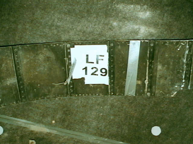
Structures 7 - LF129 - Photo 1
