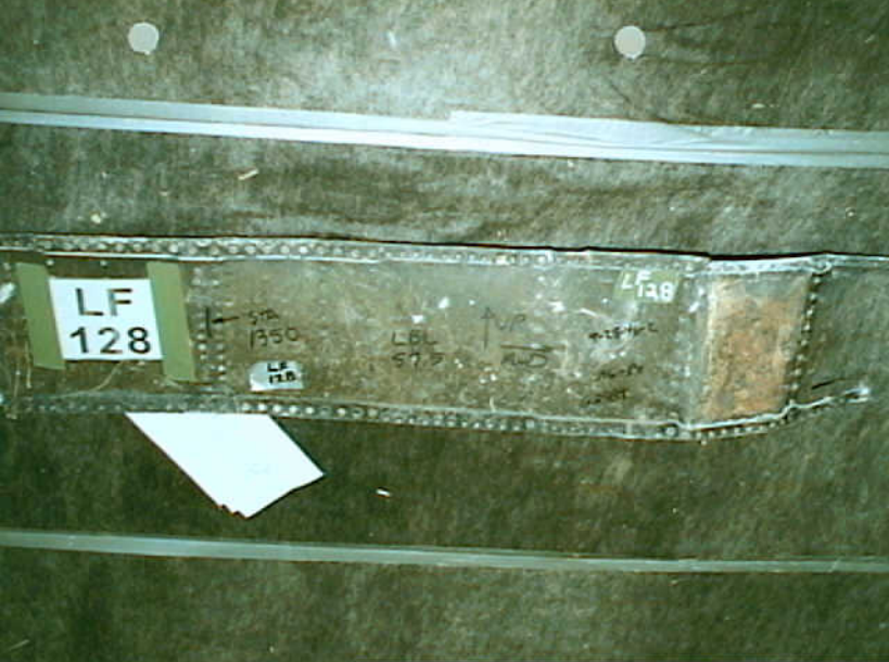
Structures 7 - LF128 - Photo 1
