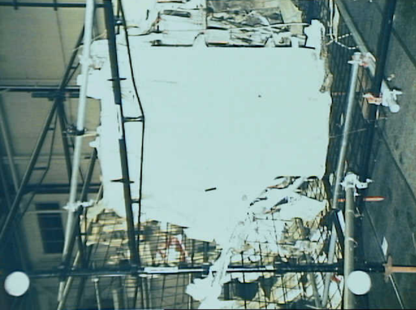
Structures 7 - LF11H - Photo 5
