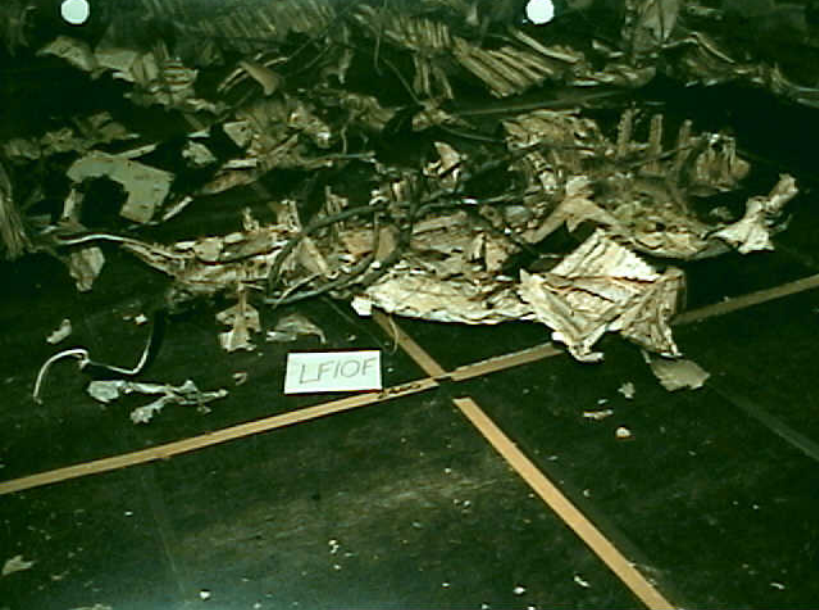
Structures 7 - LF10 - Photo 9
