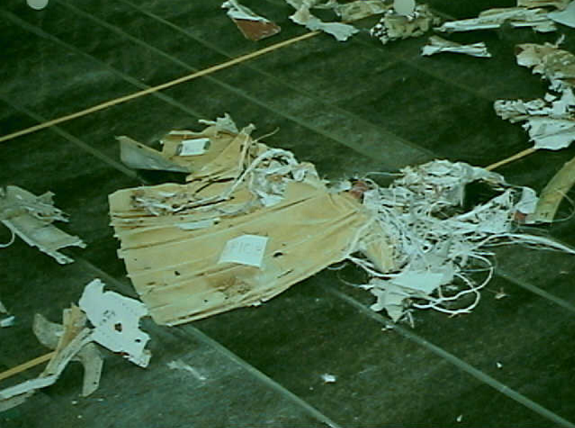
Structures 7 - LF10 - Photo 2
