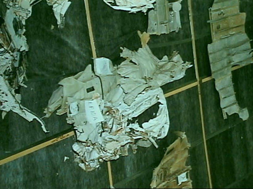
Structures 7 - LF10 - Photo 1
