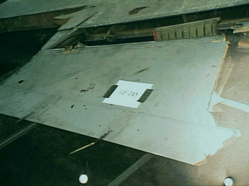
Structures 7 - LE-2D Photo 1
