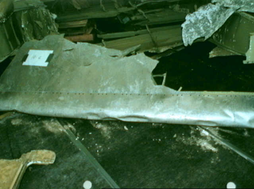
Structures 7 - H-6 Photo 1
