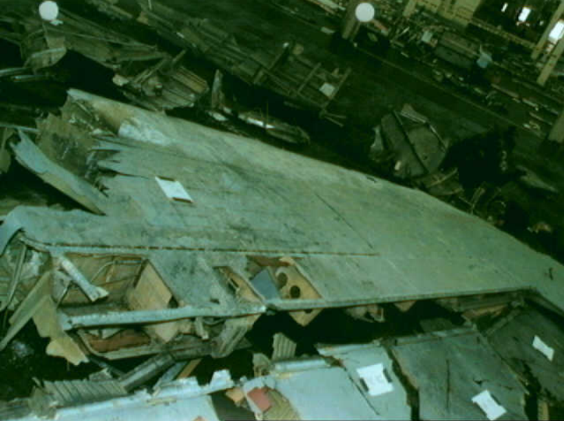
Structures 7 - H-3 Photo 1
