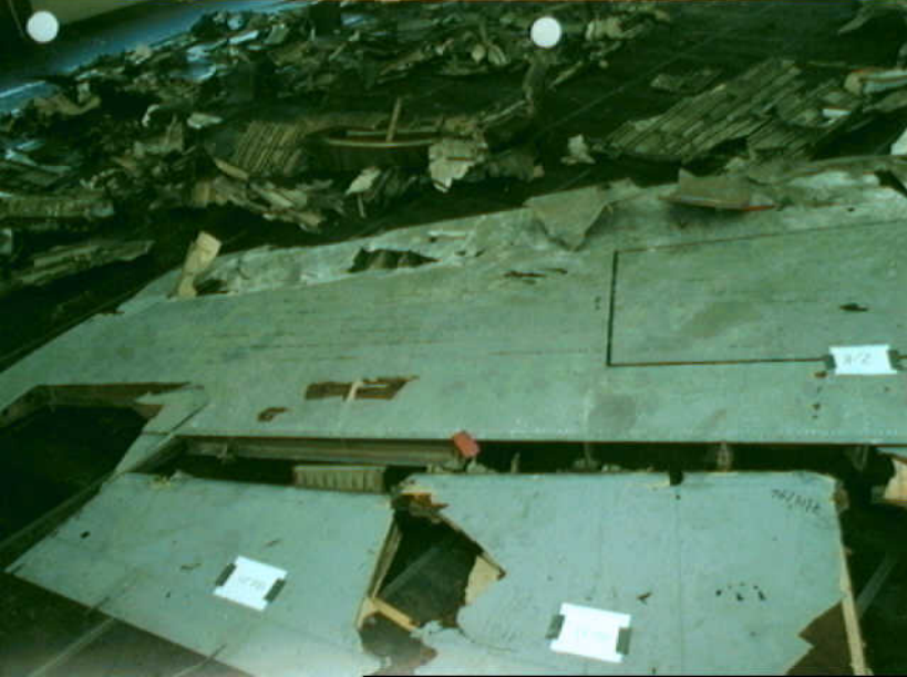
Structures 7 - H-2 Photo 4
