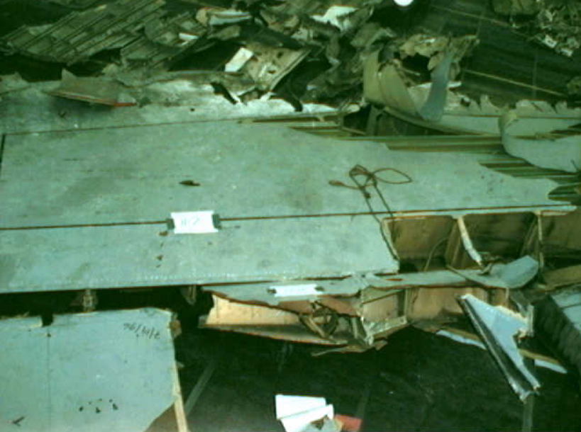
Structures 7 - H-2 Photo 3
