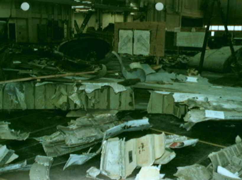
Structures 7 - H-2 Photo 2
