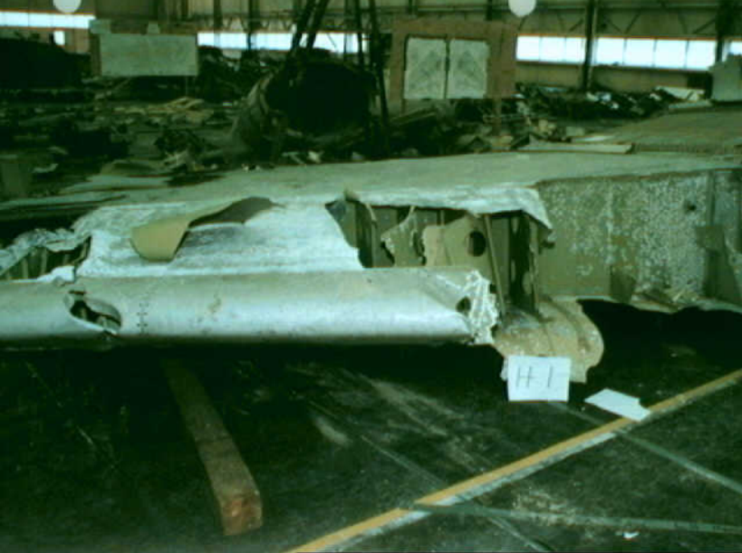
Structures 7 - H-1 Photo 7
