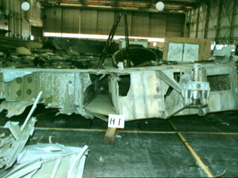
Structures 7 - H-1 Photo 6
