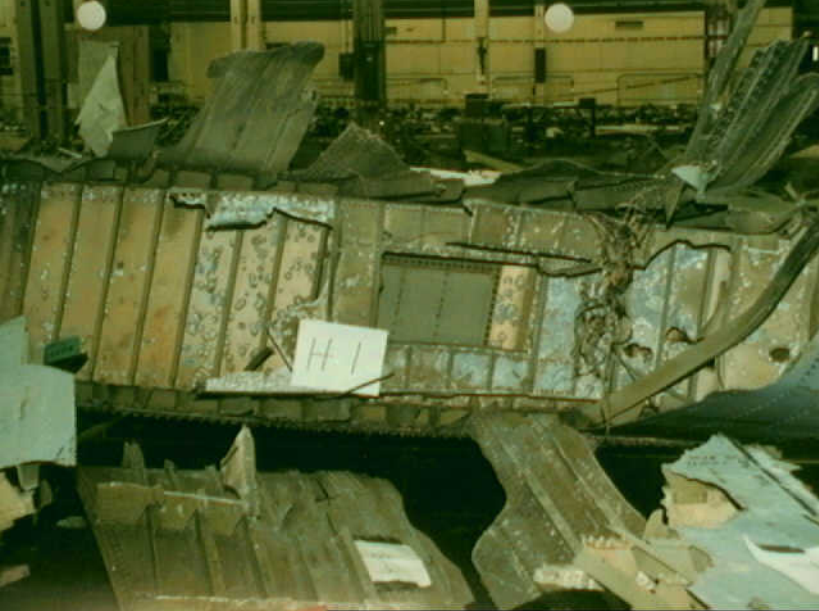
Structures 7 - H-1 Photo 2
