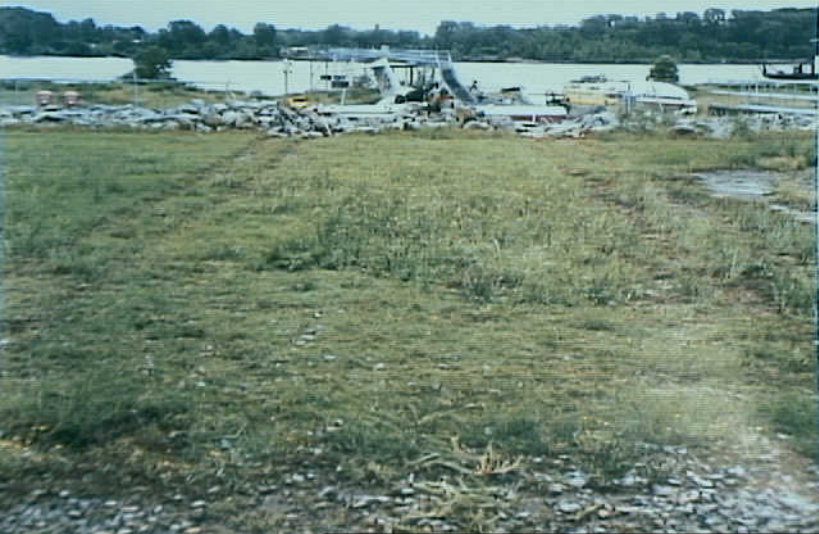
Structures 7 - Exhibit No. 7C - Photo 3. View of N215AA wreckage from runway elevation. Note the foreground tire tracks approaching the rock embankment and the subsequent drop in elevation. (Photo by J.K. Lloyd's
