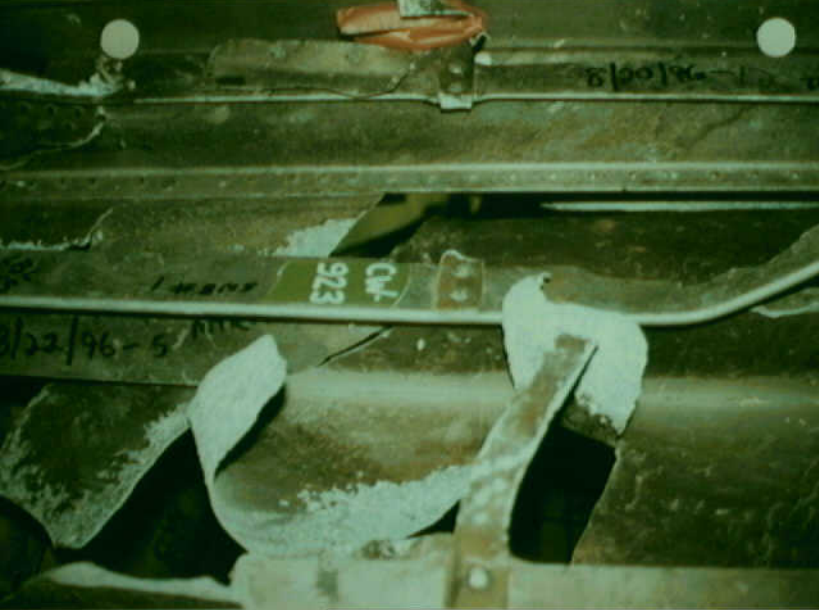
Structures 7 - CW-923 Photo 1
