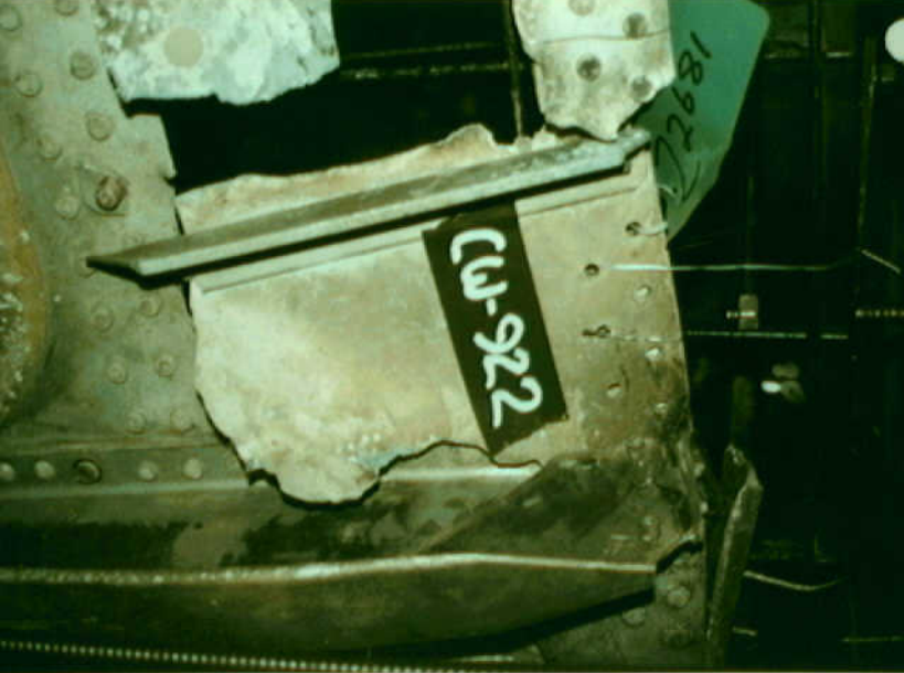
Structures 7 - CW-922 Photo 1
