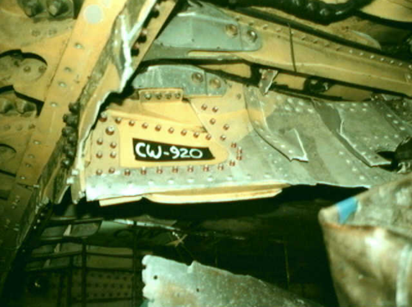
Structures 7 - CW-920 Photo 1
