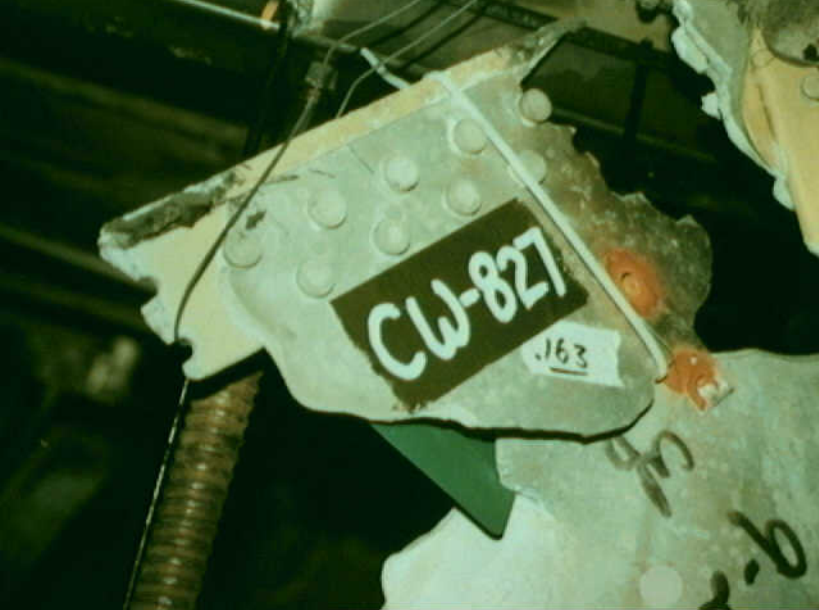
Structures 7 - CW-827 Photo 1
