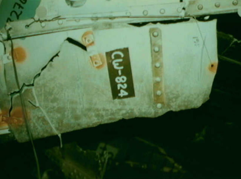
Structures 7 - CW-824 Photo 1
