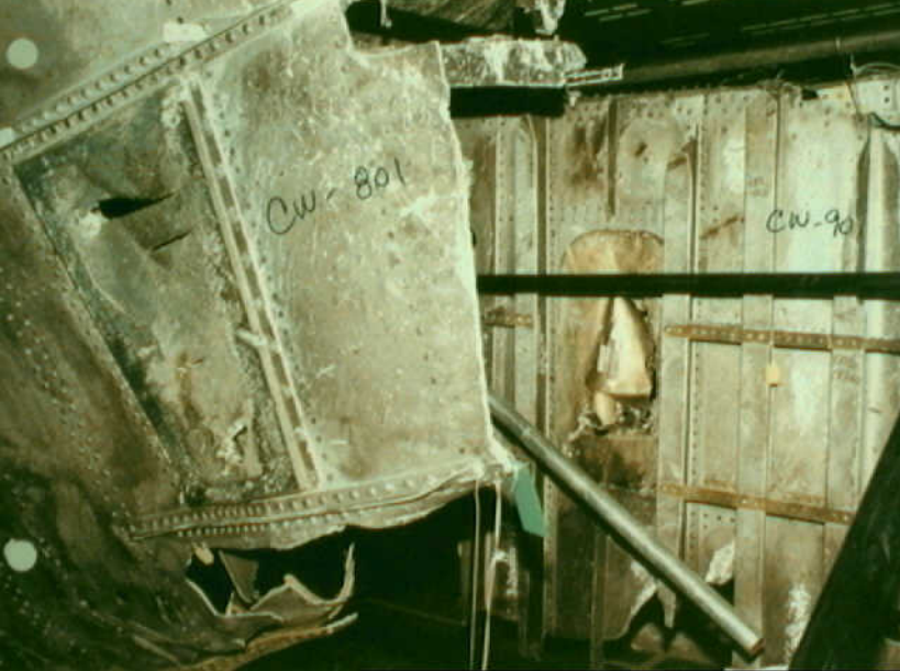
Structures 7 - CW-801 Photo 9
