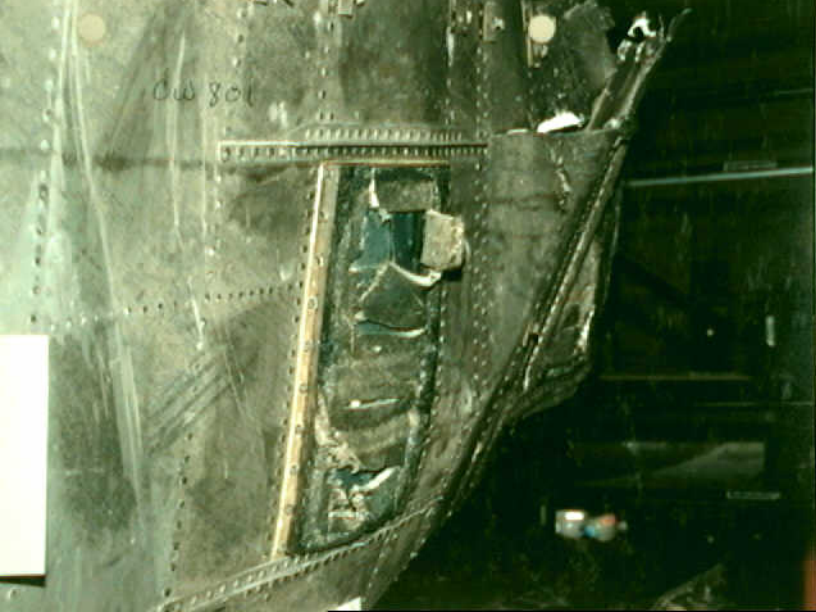
Structures 7 - CW-801 Photo 7
