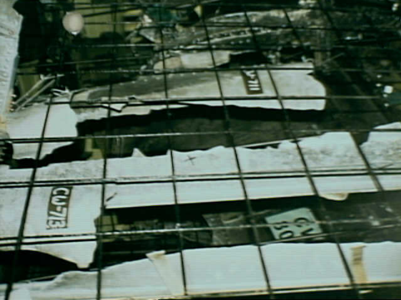
Structures 7 - CW-713 Photo 1
