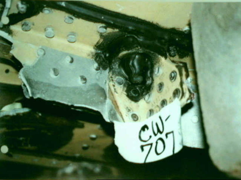
Structures 7 - CW-707 Photo 1
