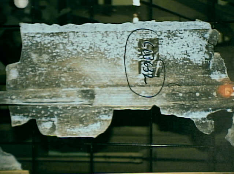
Structures 7 - CW-632 Photo 1
