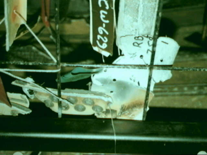
Structures 7 - CW-629 Photo 1
