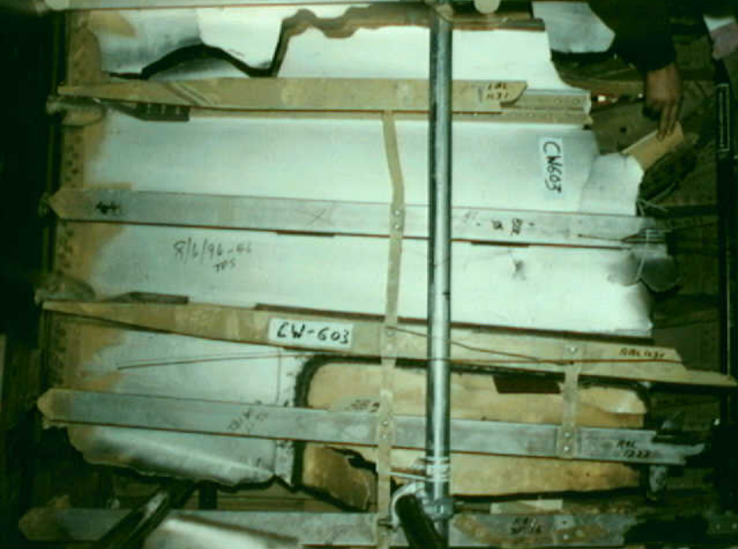
Structures 7 - CW-603 Photo 2
