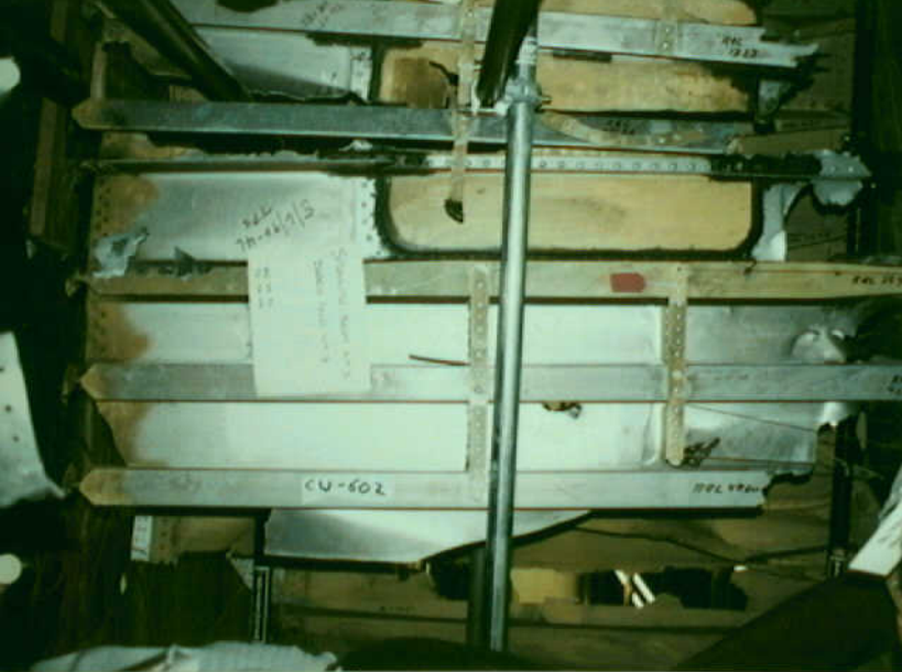
Structures 7 - CW-602 Photo 4
