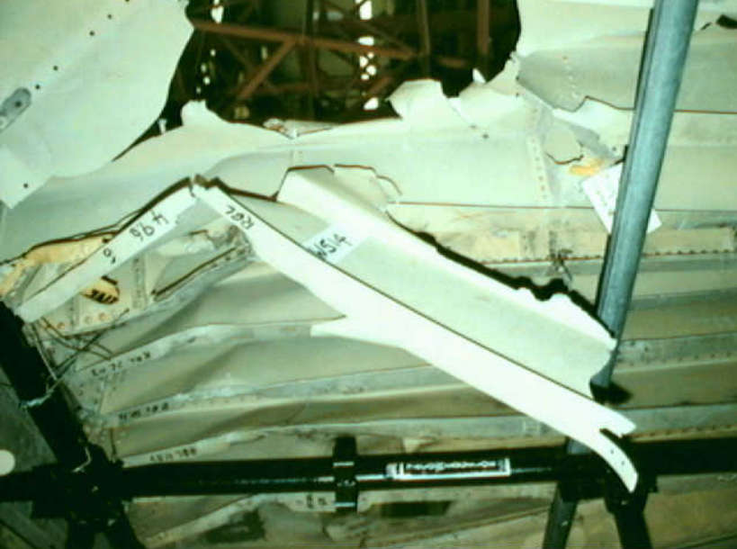
Structures 7 - CW-514 Photo 2
