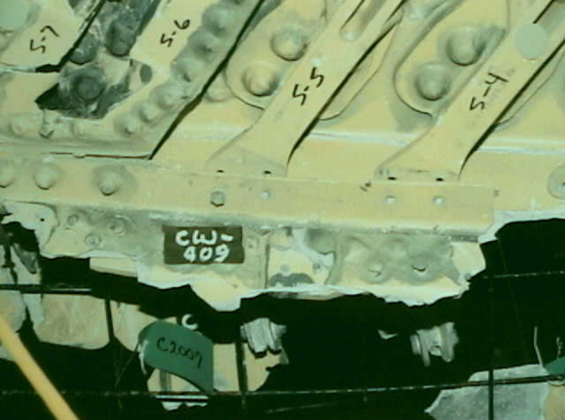
Structures 7 - CW-409 Photo 1
