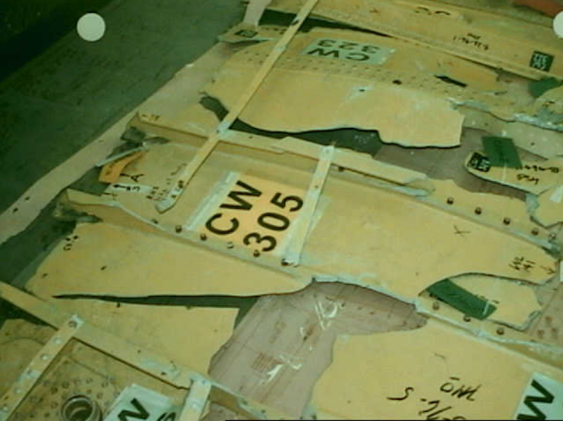
Structures 7 - CW-305 Photo 1
