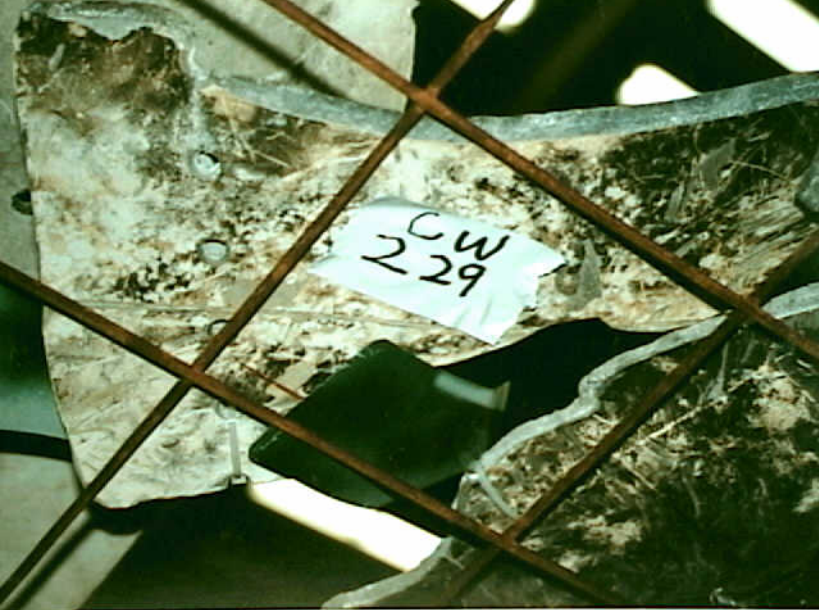
Structures 7 - CW-229 Photo 1
