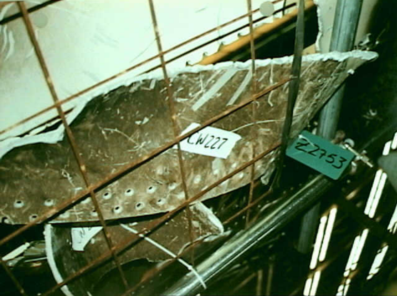
Structures 7 - CW-227 Photo 1
