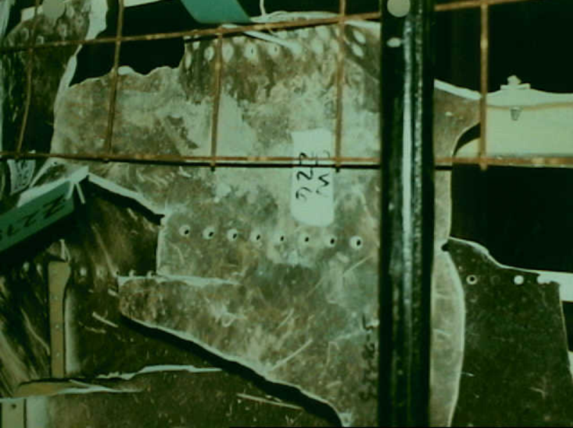
Structures 7 - CW-226 Photo 1
