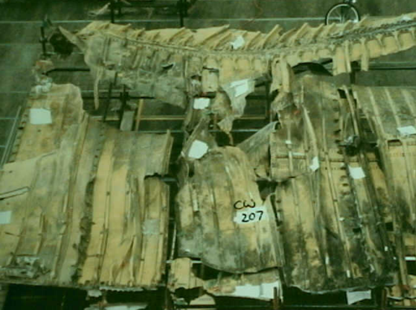
Structures 7 - CW-207 Photo 3
