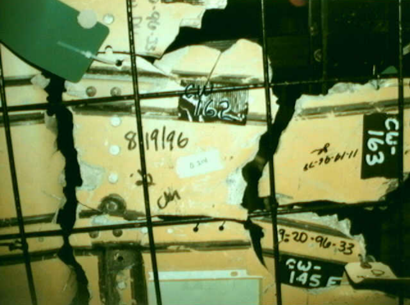
Structures 7 - CW-162 Photo 1
