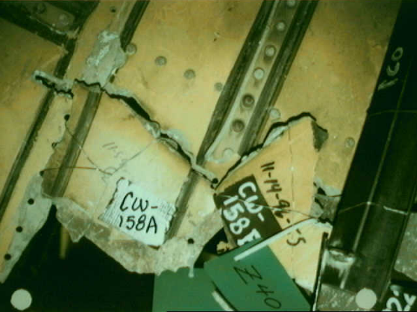
Structures 7 - CW-158AB Photo 1
