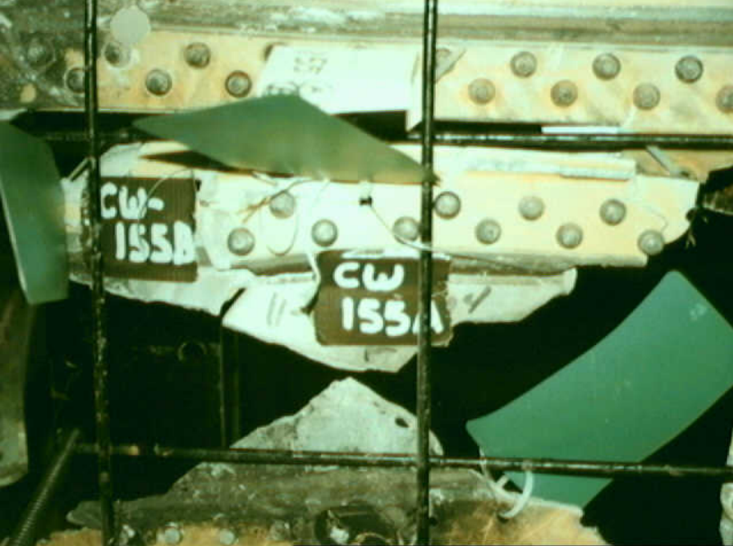
Structures 7 - CW-155A Photo 1
