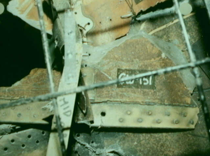
Structures 7 - CW-151 Photo 1
