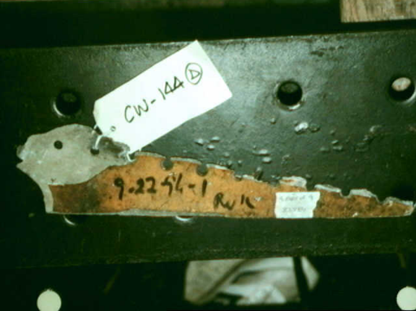
Structures 7 - CW-144D Photo 1
